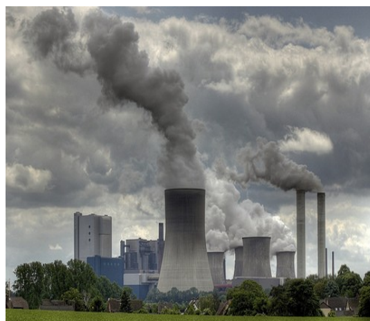
Figure 1: Coal power plant, Germany.
