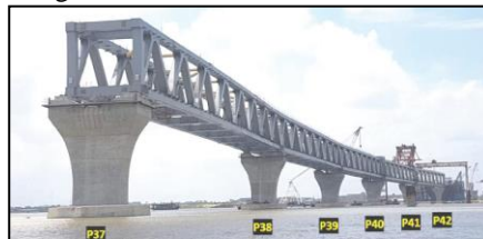
View of Padma Bridge under construction
